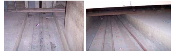
ARMOR JOINT REPAIR
