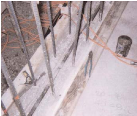
Construction waterstop joint prepared with KIM Waterstop Treatment.
